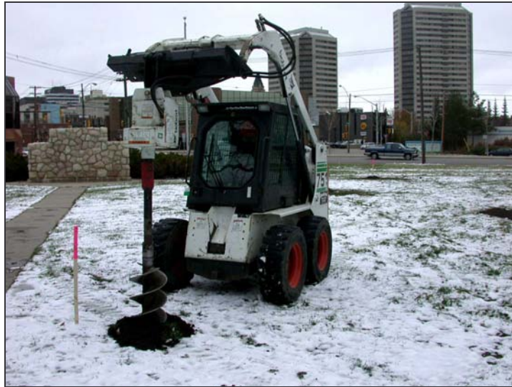
PHOTO 1 Excavating at the Gathercole Property.
